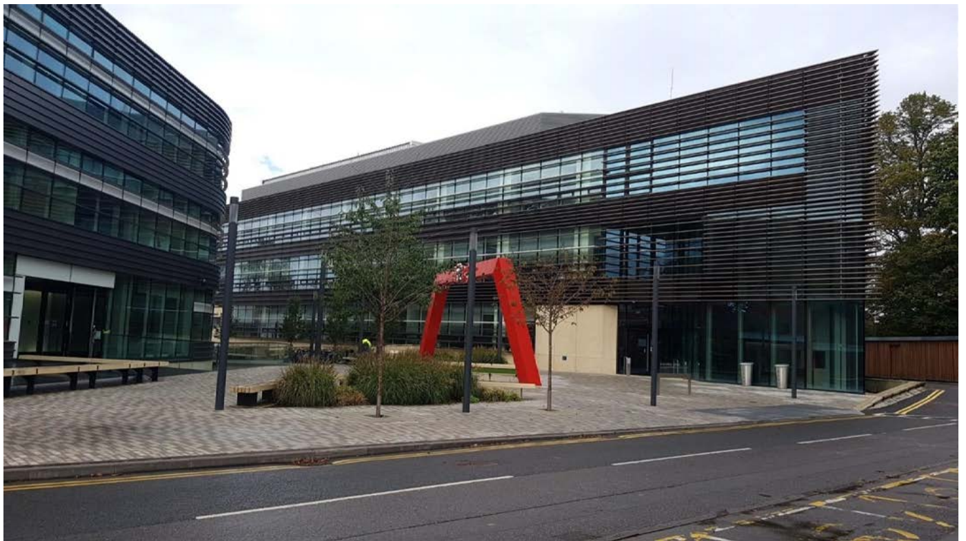
NDM Research Building
